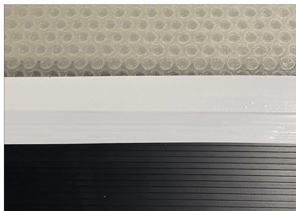
Top view - Installed Reducer Ramp with Taped Seam
