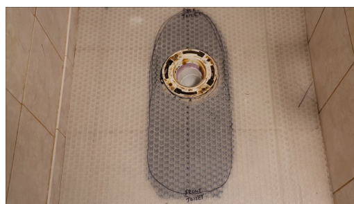
Recommended use of reinforcement around toilet mount
