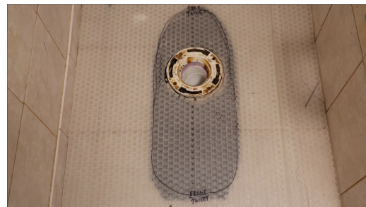
Recommended use of reinforcement around toilet mount
